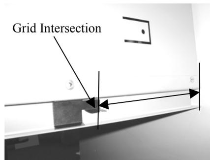
Figure 2. Clip Installation
