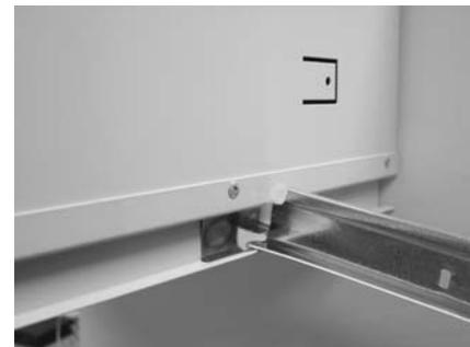
Figure 2. Grid Installation
