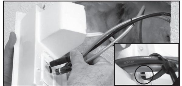
C) Slide PowerOUT panel into wall opening.
